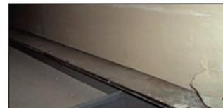
Photo 5: Joint at bottom of gypsum board has not been sealed.
