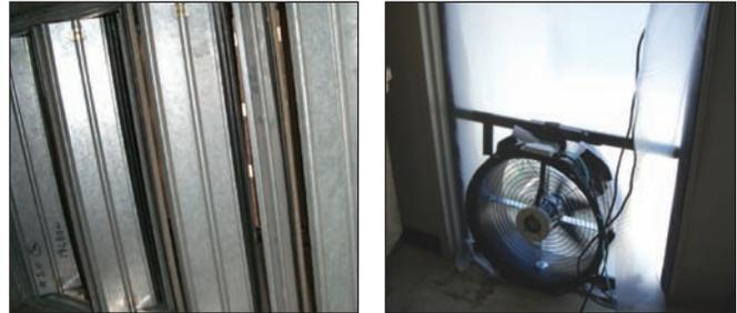
*Photo 2 (left): Relief dampers from the second floor plenum to rooftop did not close. Photo 3 (right): Blower doors installed in exterior doors.*
