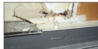
Photo 6: Sealing detail at a jog in the wall section is incomplete.
