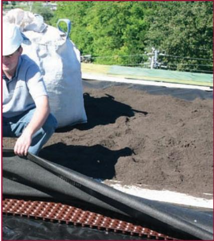
**Photo 4:** Root Barrier and Drainage Layer. Both are a big deal. Notice the filter fabric above the drainage mat and the root barrier under it.
