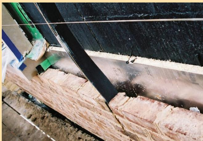
**Typical wall assembly showing continuous insulation to assist with energy-efficiency goal.**
