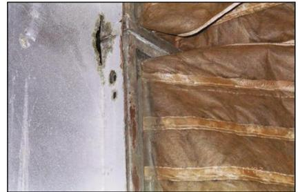
*(Left) This system serves a surgery facility in Florida. Note the filter cartridge does not even fit in the track. (Center) This photo shows disappearing filter door gasket in a college science building in San Francisco. The door is downstream of the filters and upstream of the fan. (Right) This photo shows corrosion that has caused daylight holes to outdoors as shown in this campus library unit. This hole allows bypass around the filter bank.*
